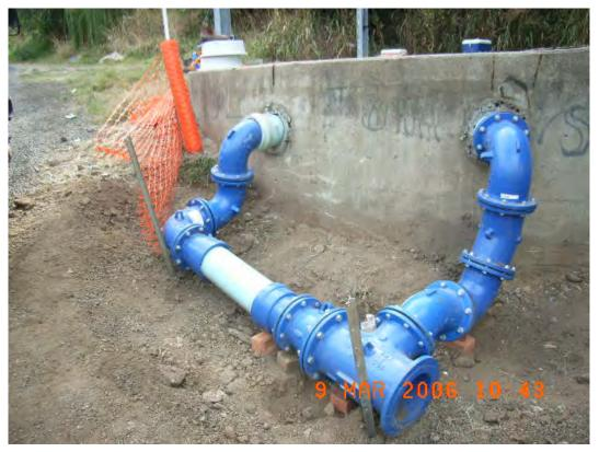
Pipework from the river well to low level pump station
