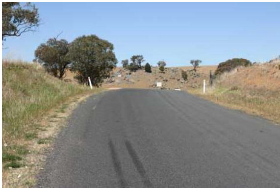
Plate 5 Reids Flat Road (view towards intersection with Battery Road) (Ref: 685_I031)
