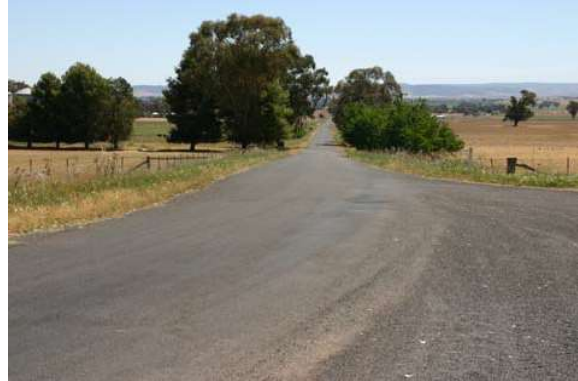
Plate 8 Morongla Road (view to intersection with Reids Flat Road) (Ref: 685_I045)
