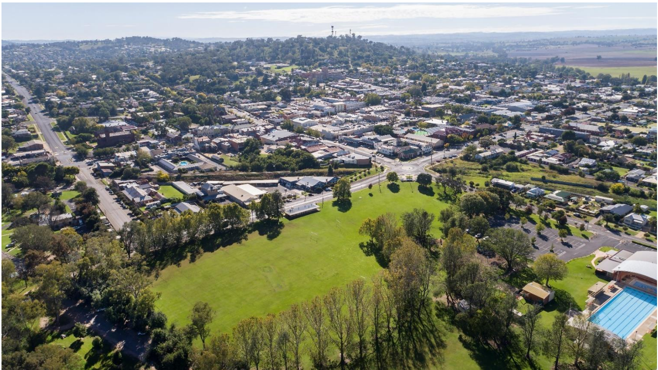
Figure 6: Aerial view of the River Park Precinct.
