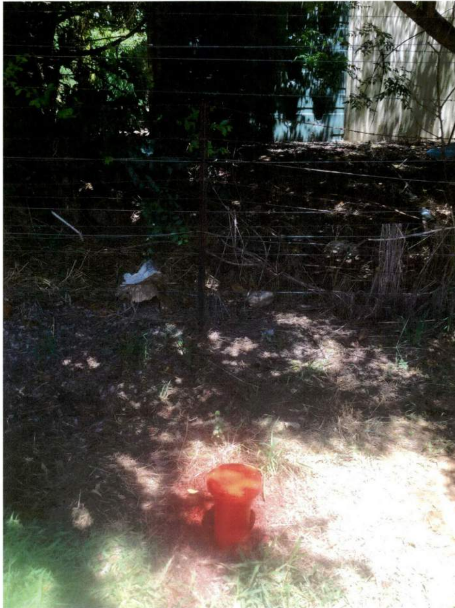
Sewer line inspection point inside 52 Grenfell Road - Walker Street storage units in background.
