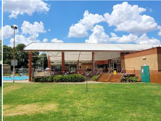
Open area where new splashpad will be constructed.
