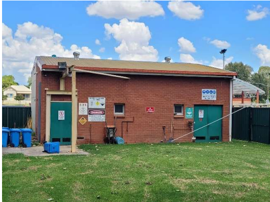
Image of existing filtration room to be demolished.
