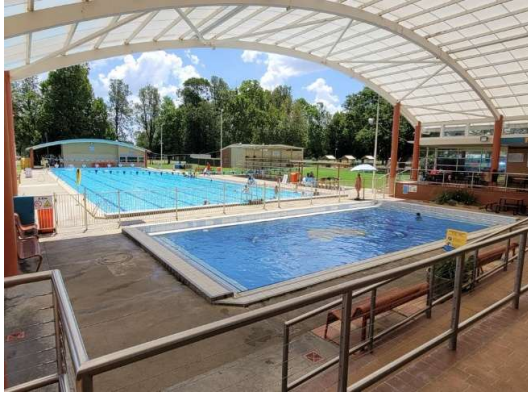
50 lap pool & program pool to be demolished and replaced with a concrete shell pool.
