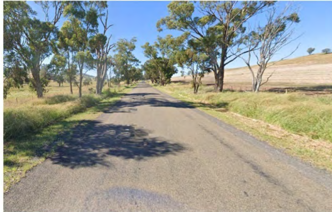
Figure 6.3: Reids Flat Road, looking south near Morongla Road
