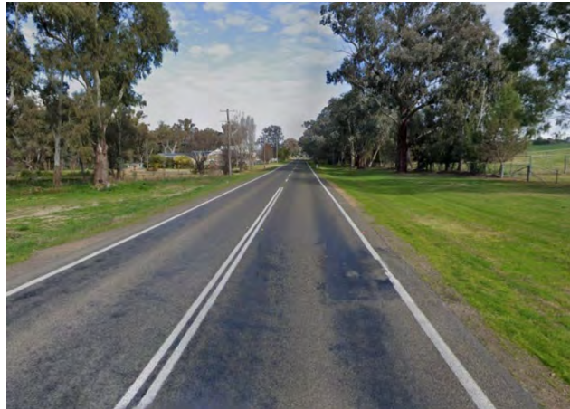
Figure 6.1: Lachlan Valley Way, looking south from the intersection with Morongla Road
