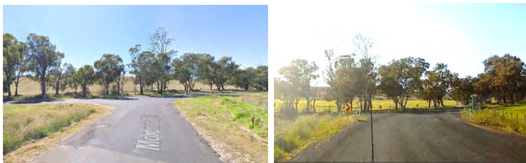
Figure 6.7: Intersection of Morongla Road & Reids Flat Road – previous (L) & upgraded (R)
